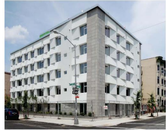
Knickerbocker Commons, the first mid-sized apartment building designed to Passive House standards in the United States
